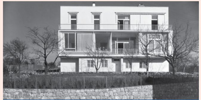
Villa Loew-Beer, Brno (architects Rudolf Baumfeld & Norbert Schlesinger). RIBA Collections
